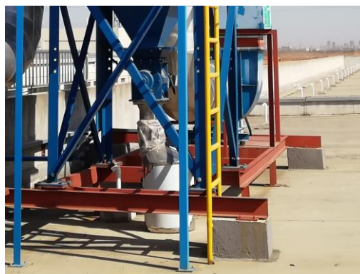
粉尘泄漏—整改后
