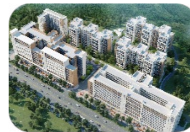
Upgraded staff dormitories
