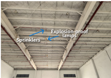
Firefighting System of the Hazardous Wastes Warehouse
